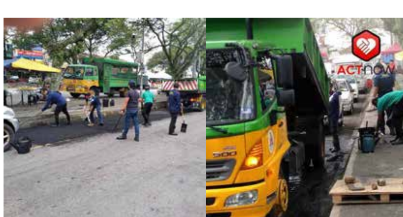
DBKL in the progress of fixing potholes
