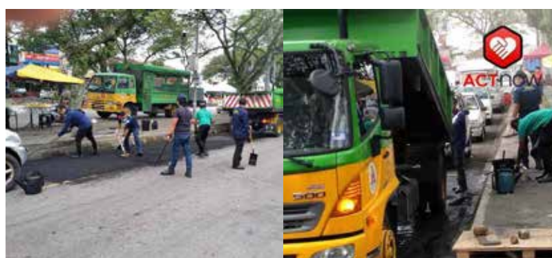
DBKL in the progress of fixing potholes
